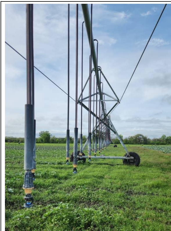
Photo 5-1 Pivot irrigation system employed by the Proponent (photo: A Blume)
