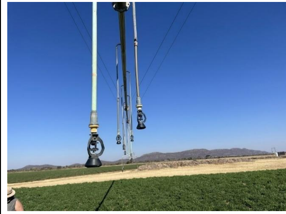
Photo 4-35 Typical emitters used by the centre pivot system
