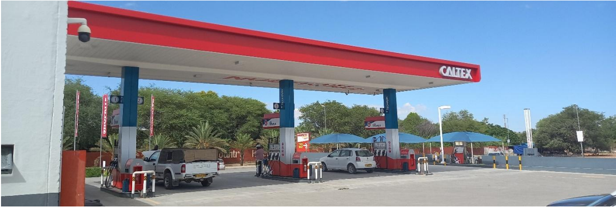
Figure 6: Pumps under a canopy and on an elevated Island
