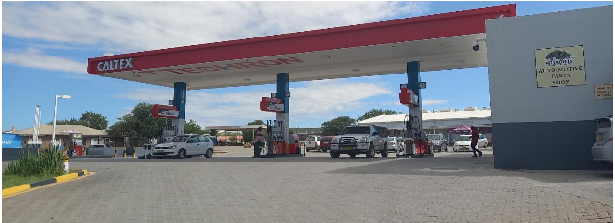
Figure 3: FRO seen from South to North
