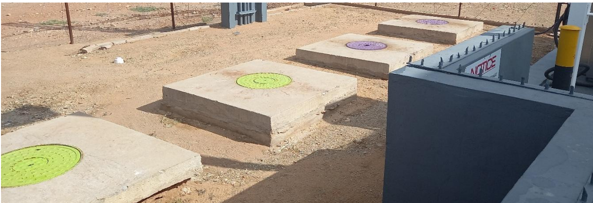
Figure 8: USTs two per ULP and ADO
