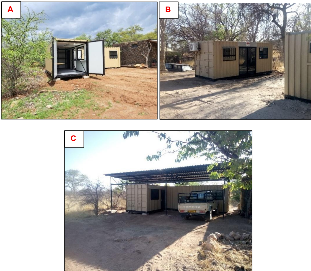
Figure 2-5: The Okomutati Base Camp workshop (A) and storeroom containers, and (B) the office and boardroom container, as well as the shade structure built in October 2025 (C)
