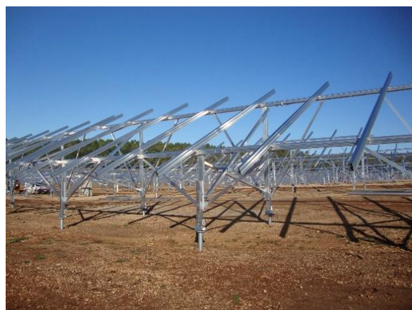
Photo 5-1 Typical anodised aluminium frame
