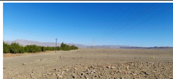
Photo 5-6 Existing power line connecting to the substation
