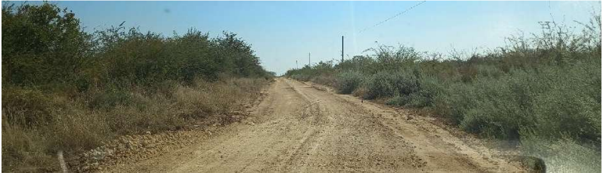
Figure 4: Access road to the borrow pit
