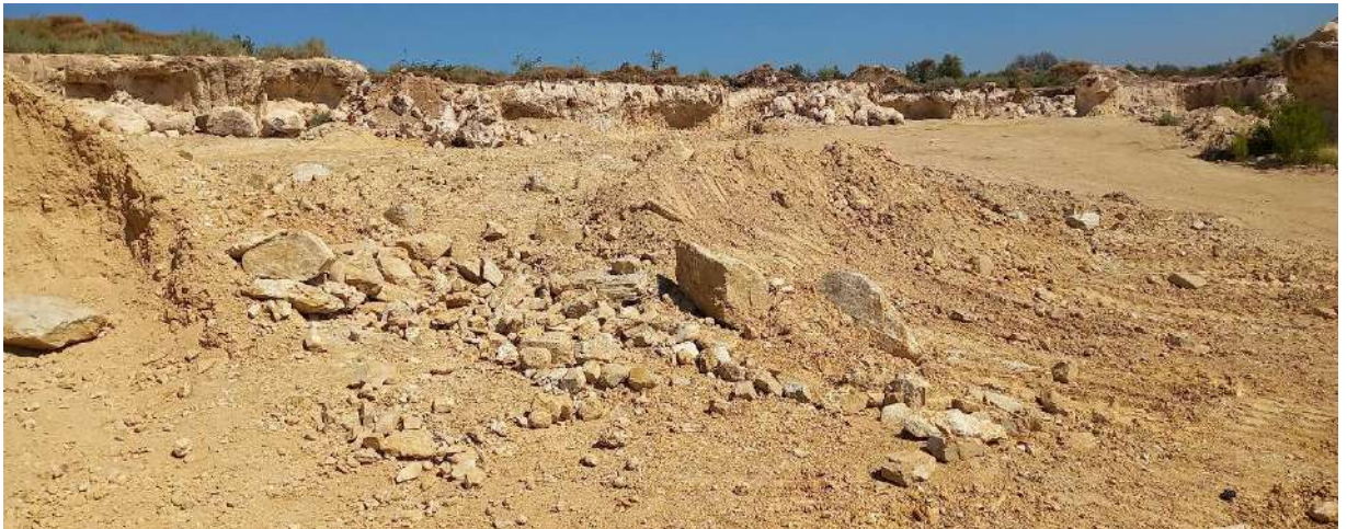
Figure 6: View of the borrow pit to the west
