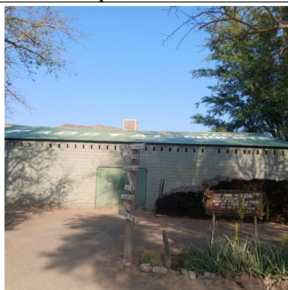
Photo 3-6 Old farm stall now used as storage shed
