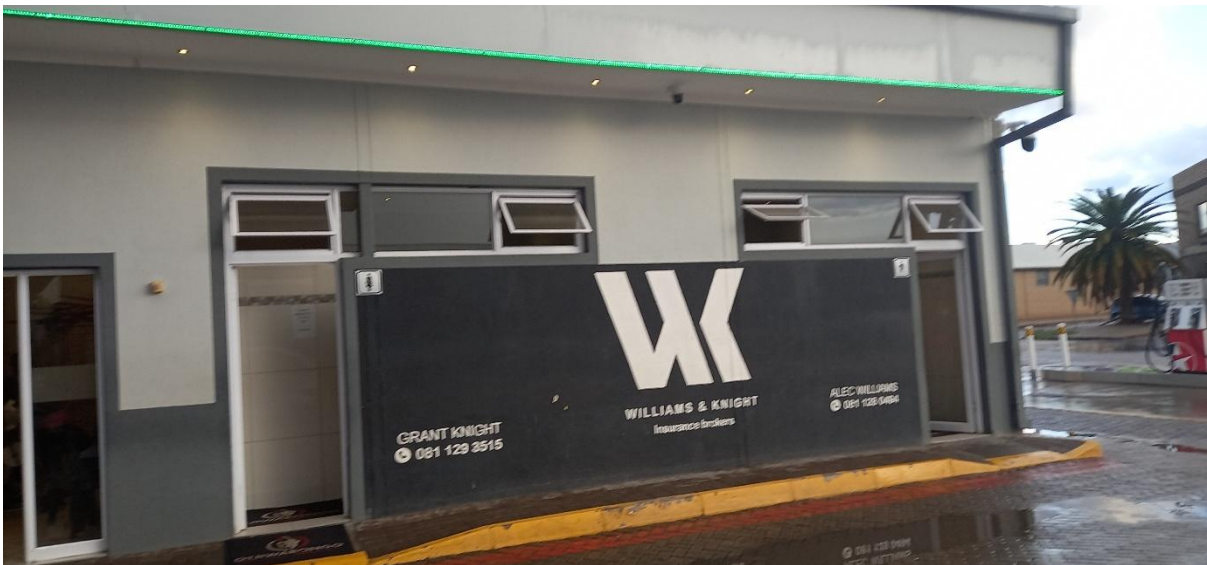
Figure 15: Toilet facilities at Caltex
