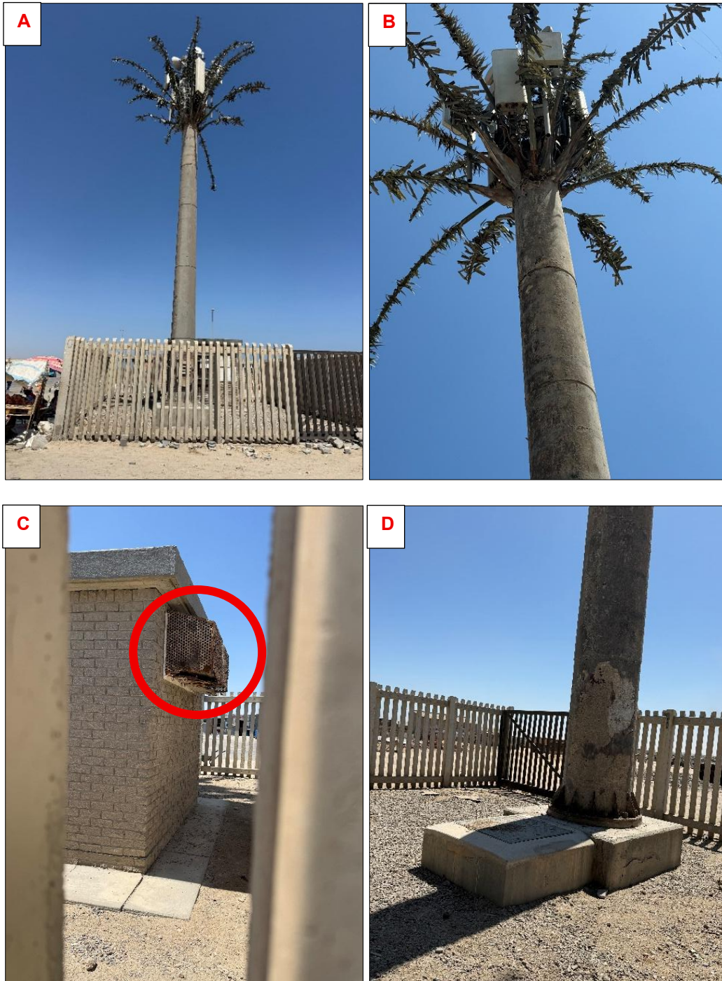
Figure 1-3: Photos of the current (dilapidated) status of the DRC tower site: A- The fenced monopole tower and support infrastructure; B- Top part of the tower with artificial leaves/branches and rectangular boxes with antennae; C-The dilapidated status of the cabinet ventilation of the DRC tower site; D- The dilapidated tower base foundation
