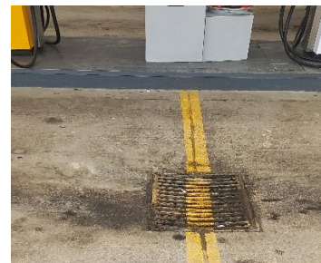
Figure 11: Forecourt runoff water drainage channel
