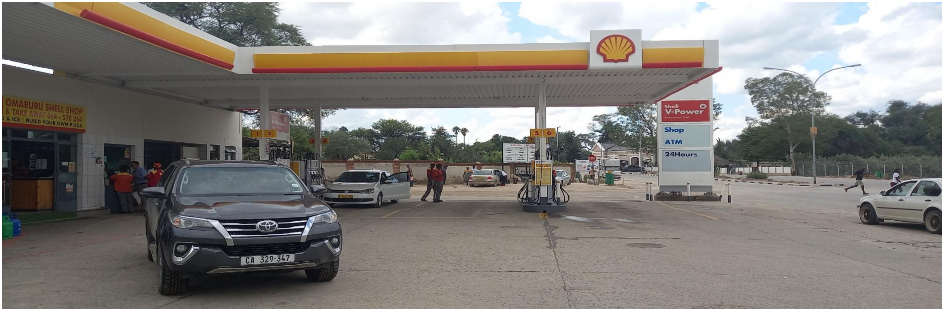
Figure 3: OEW Shell service Station seen from West to East
