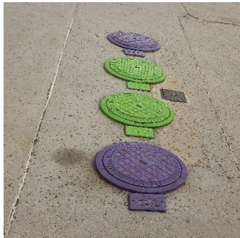
Figure 6: Colour coded USTs
