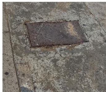
Figure 13: Manhole cover for the runoff water storage chamber
