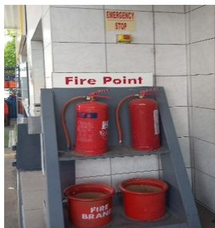
Figure 12: Fire extinguishers & spill cleaning sand
