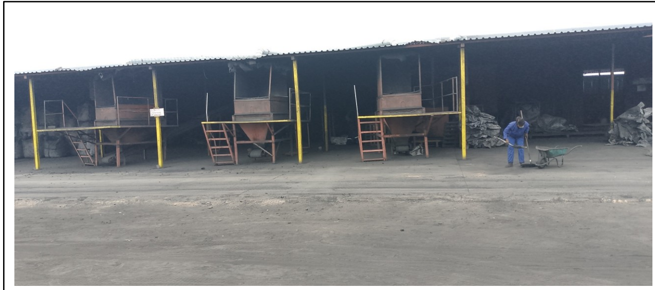
c) Housekeeping around the screening area
