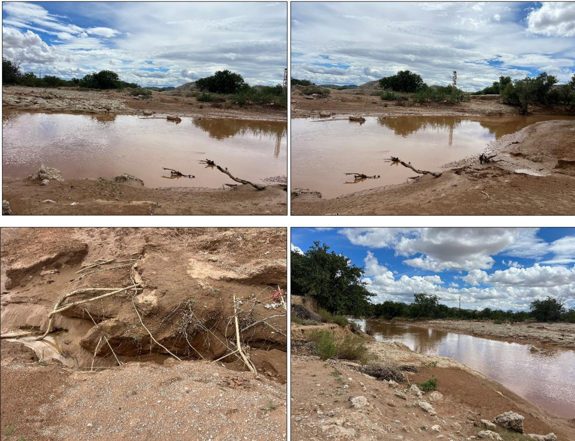
Figure 2-1: The condition of the DR3703-Oute River site for the bridge construction in March 2026
