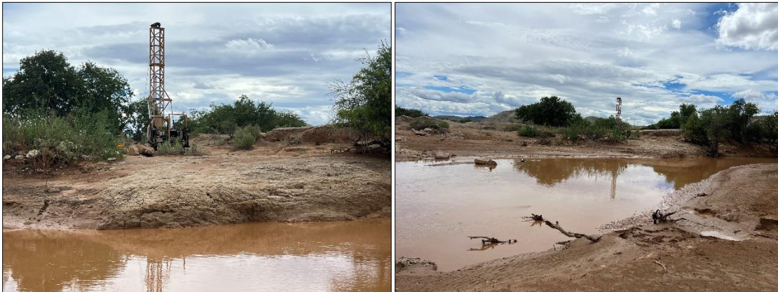
Figure 2-2: The ongoing project’s geotechnical investigation (geotechnical drilling) in March 2026
