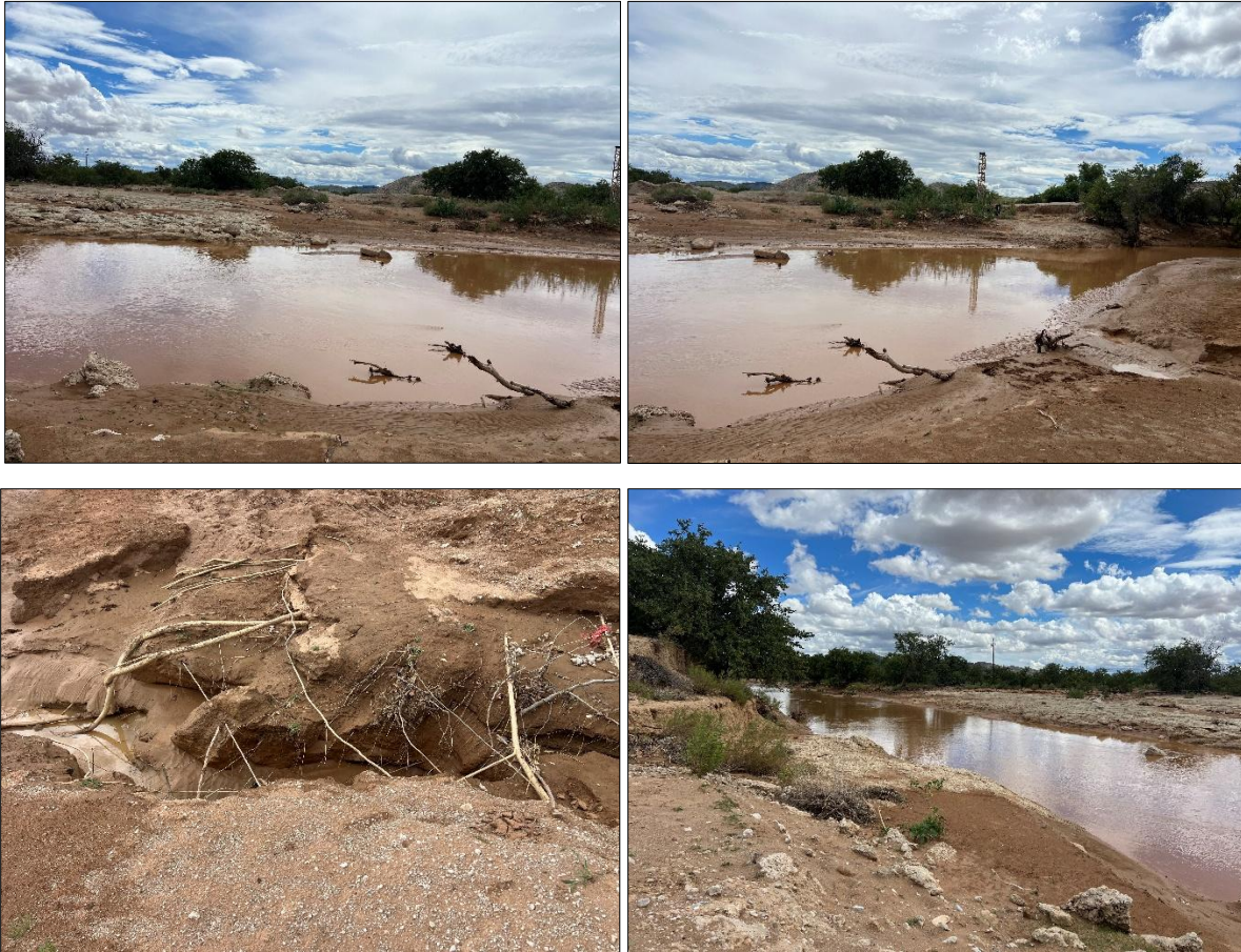
Figure 2-1: The condition of the DR3703-Oute River site for the bridge construction in March 2026
