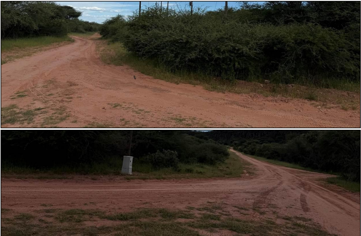
Figure 11: Gravel access Road to the Project Site
