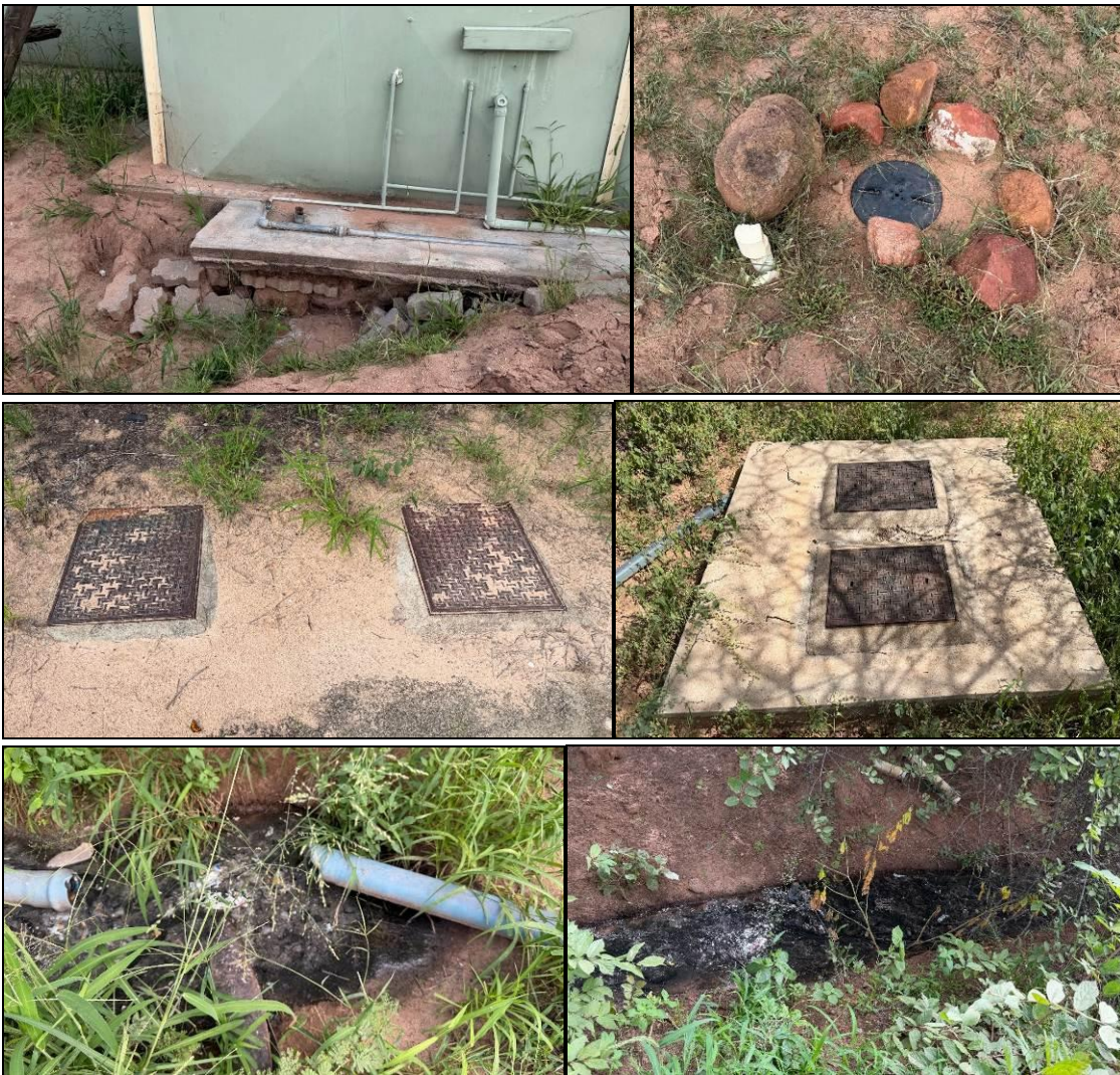
Figure 2: Existing sewer infrastructure present on site
