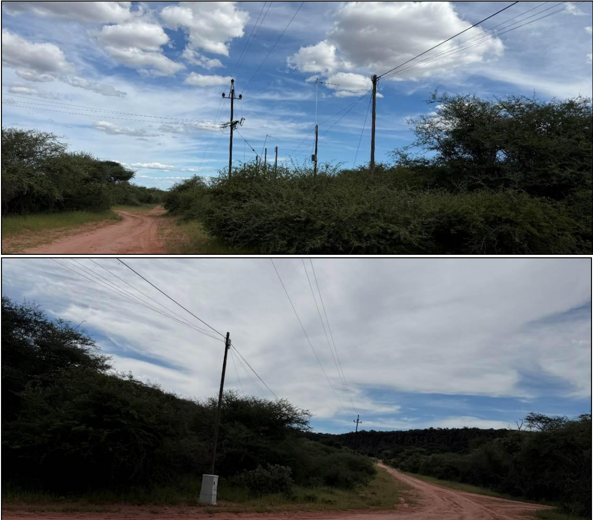
Figure 12: Electricity Powerline providing power to the Project Site
