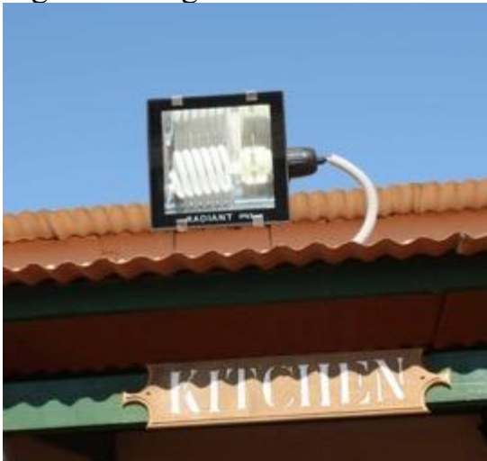
Figure 12: Light Fixture Removed
