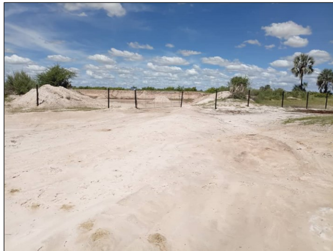
Figure 2: Emono borrow pit site (fenced off).
