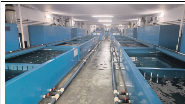
Photo 4-7 Holding tanks at the processing plant
