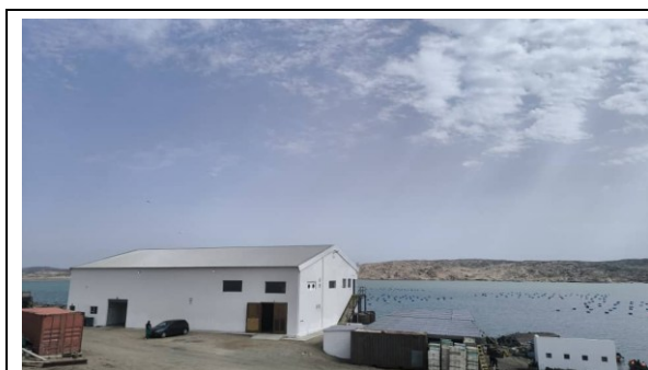
Photo 4-5 Processing plant from the outside
