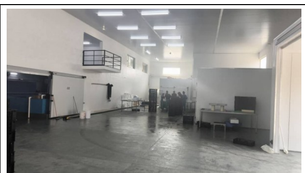
Photo 4-6 Interior of the processing plant
