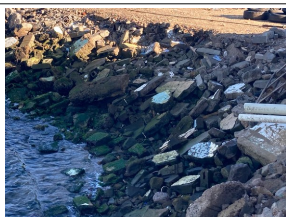
Photo 4-12 Seawater discharge point
