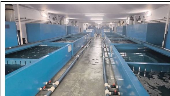
Photo 4-7 Holding tanks at the processing plant
