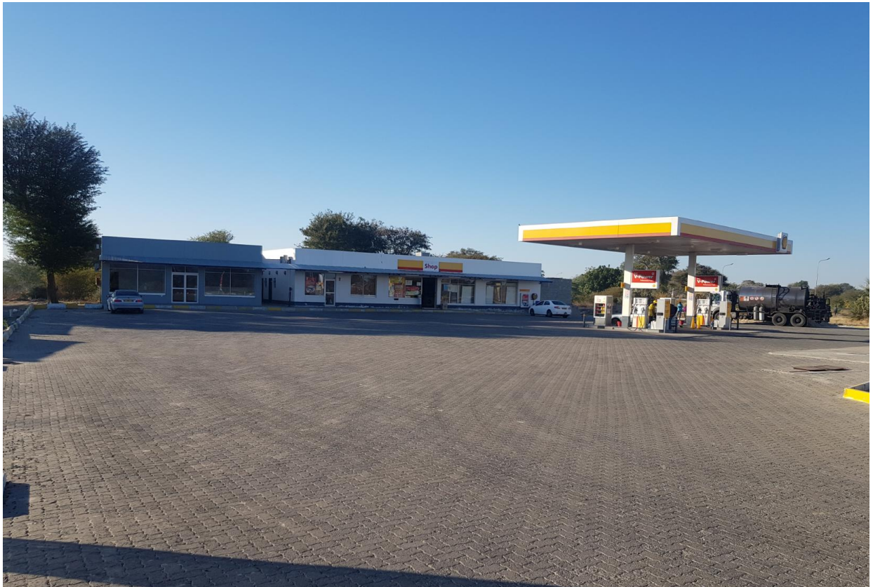
Photo 1. The existing Bukalo Service Centre .
