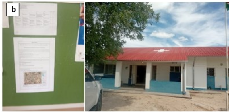
Site Notices at Tsandi Constituency Office (a) and Onamandongo Clinic (b)
