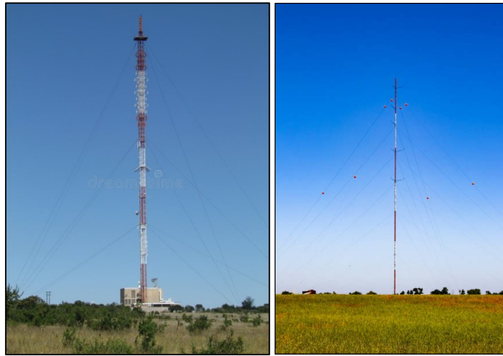
Figure 2: Typical red and white painted Guyed Mast tower structures
