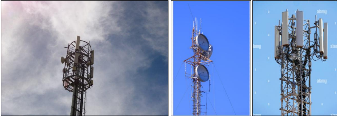
Figure 2-2: Different types of panel-type antennae
