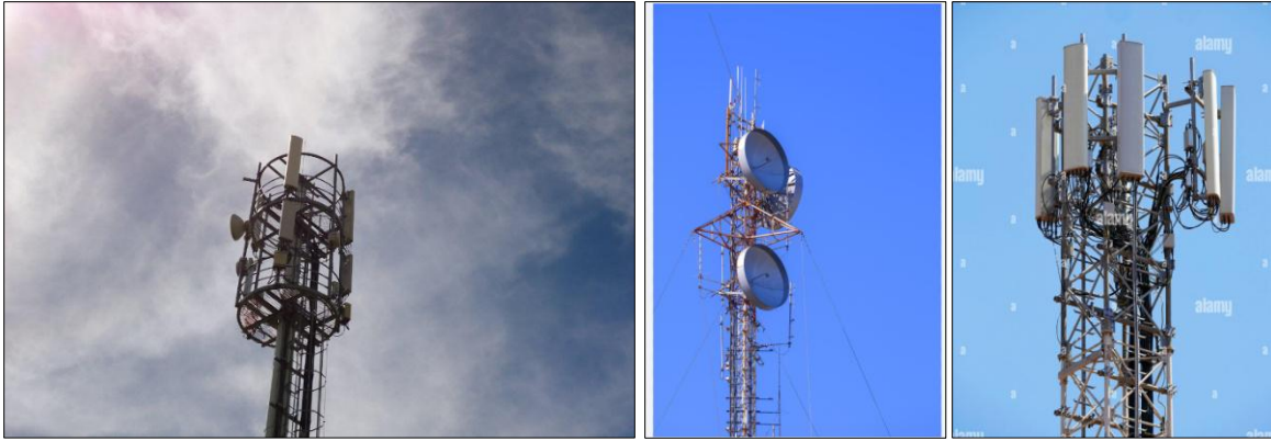
Figure 2-2: Different types of panel-type antennae
