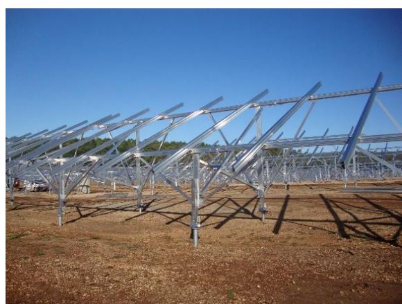
Photo 5-1 Typical anodized aluminium frame
