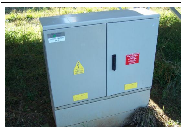
Photo 5-3 Typical array enclosure
