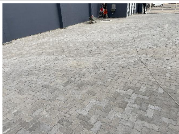
Photo 4-5 Heavy duty interlocks on the exterior of the warehouse
