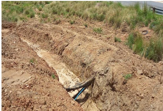
Figure 10: Exposed Electrical Cables at the Project Site
