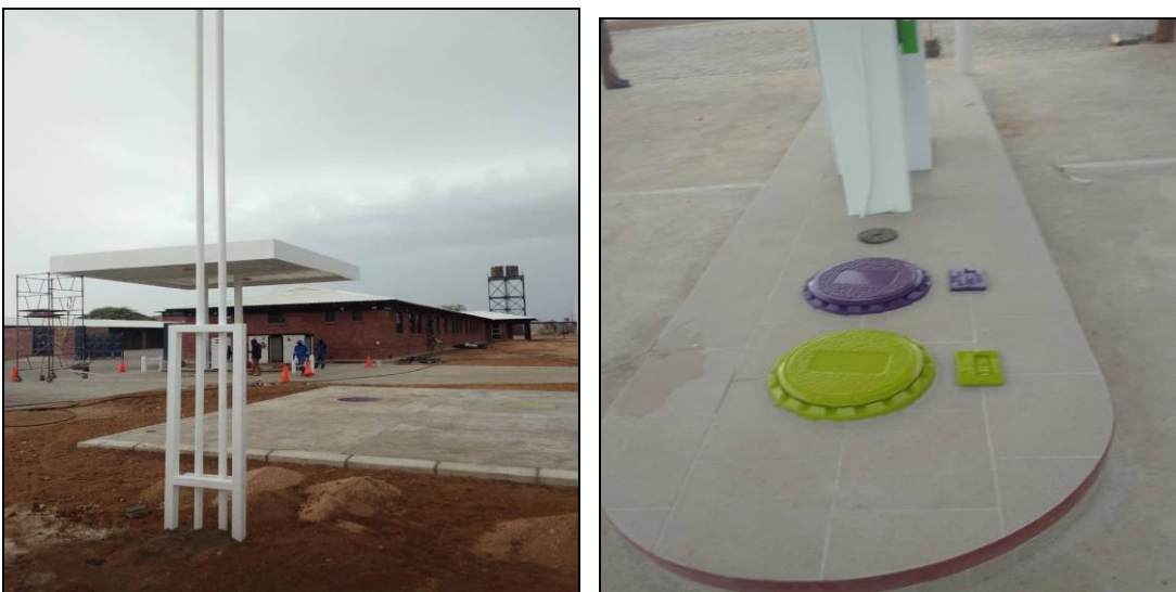
Figure 11: The RC Spill Slab
