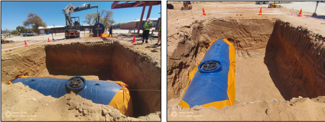
Figure 6: During the construction of the facility
