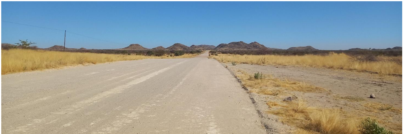
Figure 3: View to the North from the T-junction
