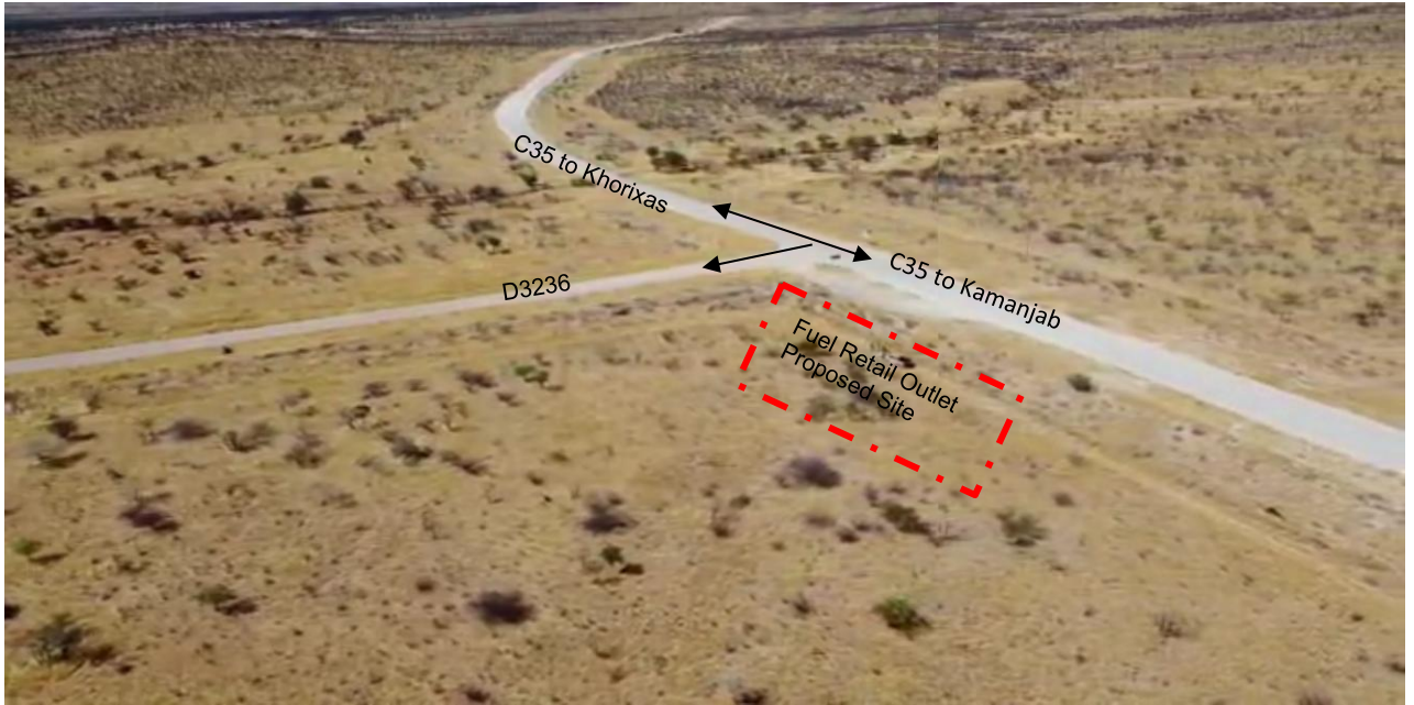
Figure 2: An Aerial View of the Project Site - Corner of C35 and D3236
