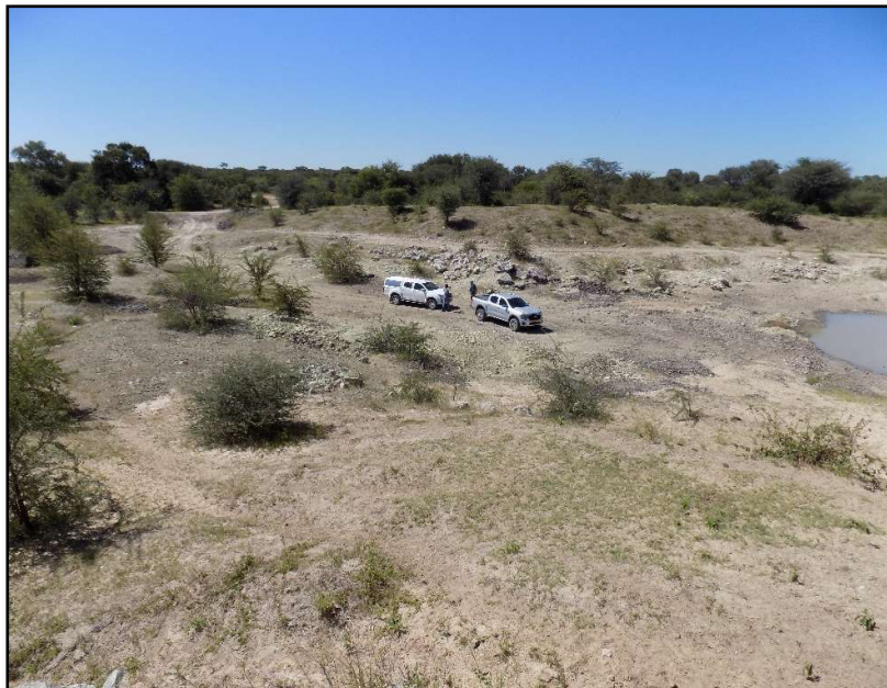
Figure 3. Photo of the current activities present in the borrow pit km 91.
