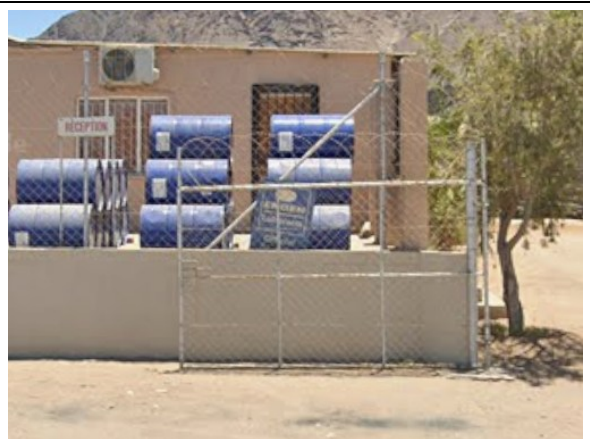
Photo 4-4 Office building with oil drums (Google Maps, 2025)
