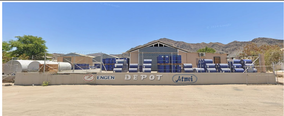
Photo 4-5 Google Street view of the warehouse and fuel tanks (Google Maps, 2025)
