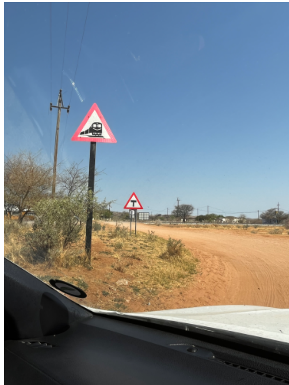
Three Phase Electrical Lines to site
