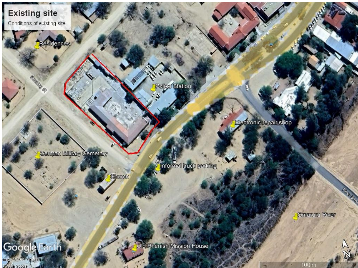
Figure 6: Land use characteristics of the site
