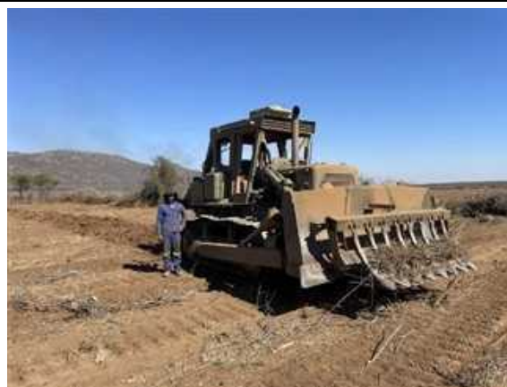
Photo 4-8 Land clearing machine and operator
