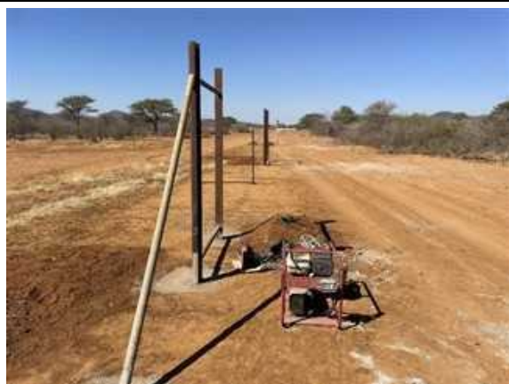
Photo 4-7 Construction of the Farm fence
