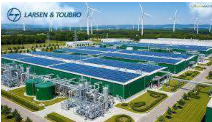
Figure 2: Larsen & Toubro Green Hydrogen Plant in India
