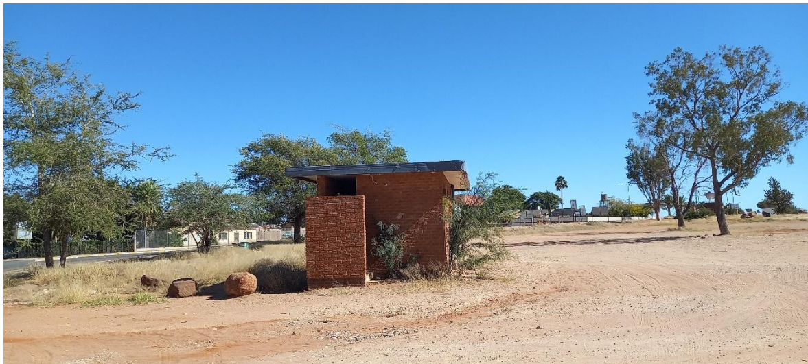
Figure 6: A public Sanitation Facility on the property (Erf 1587)
