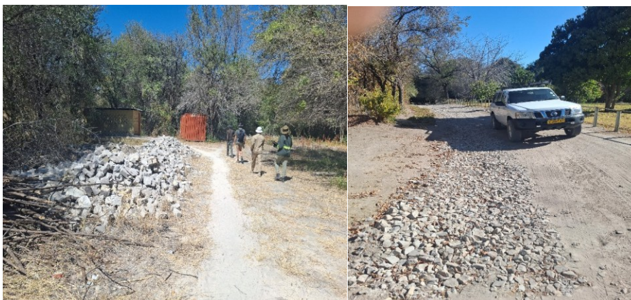
Figure 11: LHS building rubble for road repair and RHS eroded roads repaired with building rubble.
