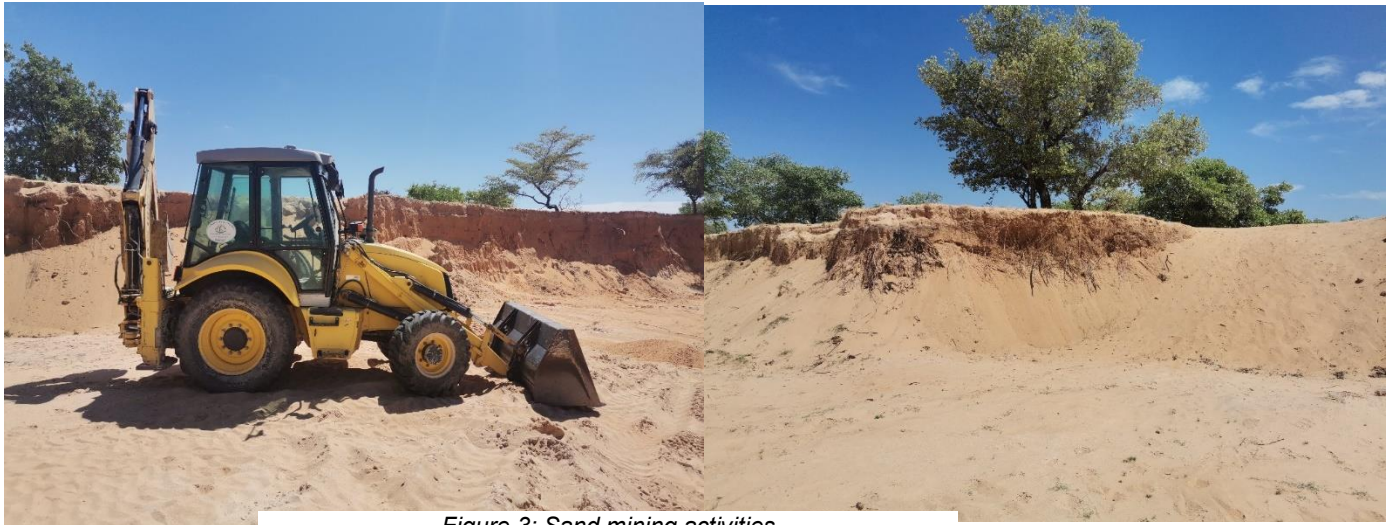
Figure 3: Sand mining activities
