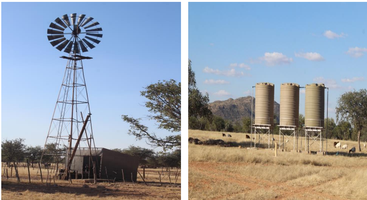
Figure 3: Existing water infrastructures in the area.
