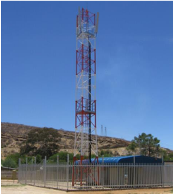
Figure 3: Typical 30-meter lattice telecommunication tower structure and form (visual purposes only)
