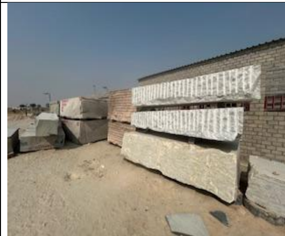
Receiving of stone blocks
