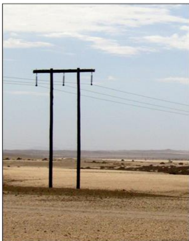
Figure 5.1. a) Structure for the intermediate pole for the proposed new Omburu-Omaruru 44 kV overhead line; b) technical diagram showing earthing system (above red) and an example of the structure in the Erongo region (below).
