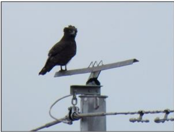
Figure 9.5. Example of a Brown Snake Eagle making use of a perching structure fitted to the top of a 66 kV steel monopole.
