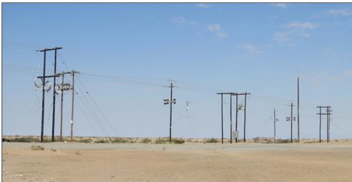
Figure 5.2. Typical transformer/step-down structures for low/medium voltage overhead line structures; note the higher H-pole on the left, used for extra strength (and height, e.g. at road crossings).
