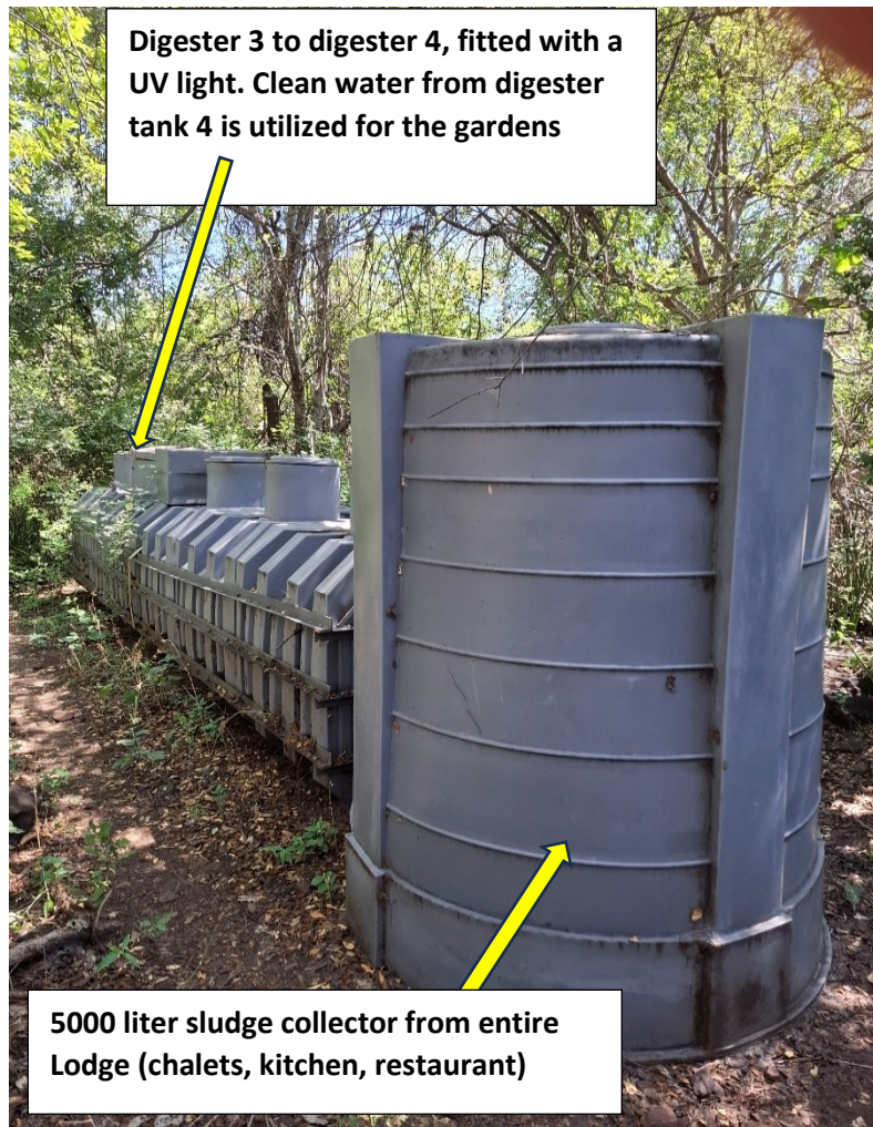
Figure 6: Example of the 4-compartment digester for grey and black water; the sludge proceeds through each septic tank with an UV light attached between digester 3 to digester 4 .
