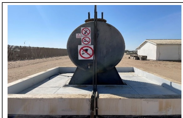
Photo 3-12 Diesel tank for backup generators
