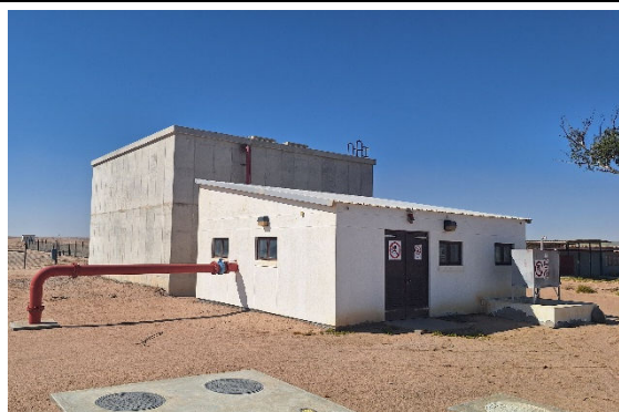
Photo 3-9 Water reservoir and pump room
