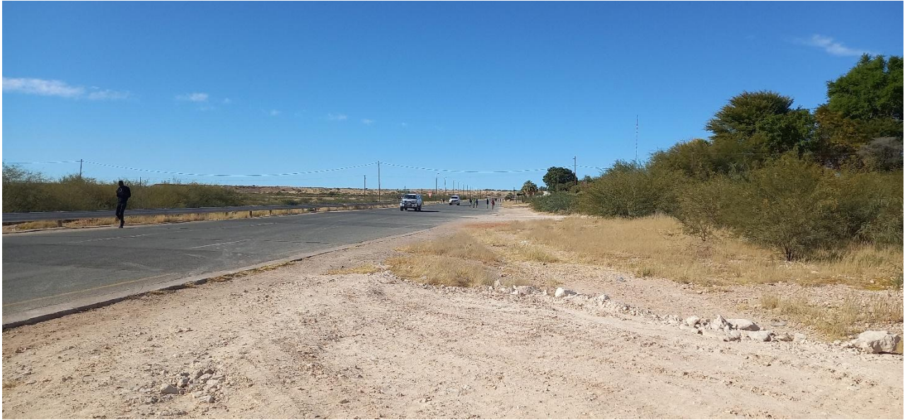
Figure 7: View to the East along Adjacent C20 Leading towards Aranos-Gobabis
