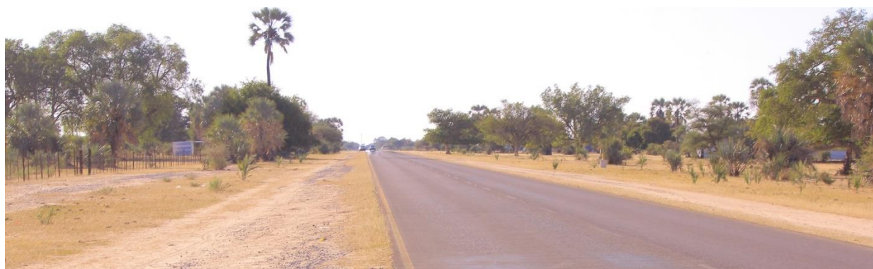
Figure 10: Road infrastructure in Ohangwena,
