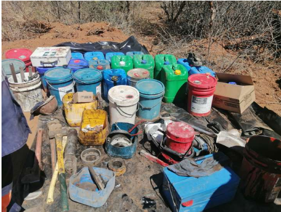
Figure 6 - All material and tools stored on a PVC lined ground to prevent soil contamination in the event of spillage
