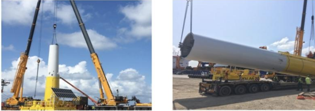
Figure 4: Installation of Lower Tower (DotPower, 2025)
