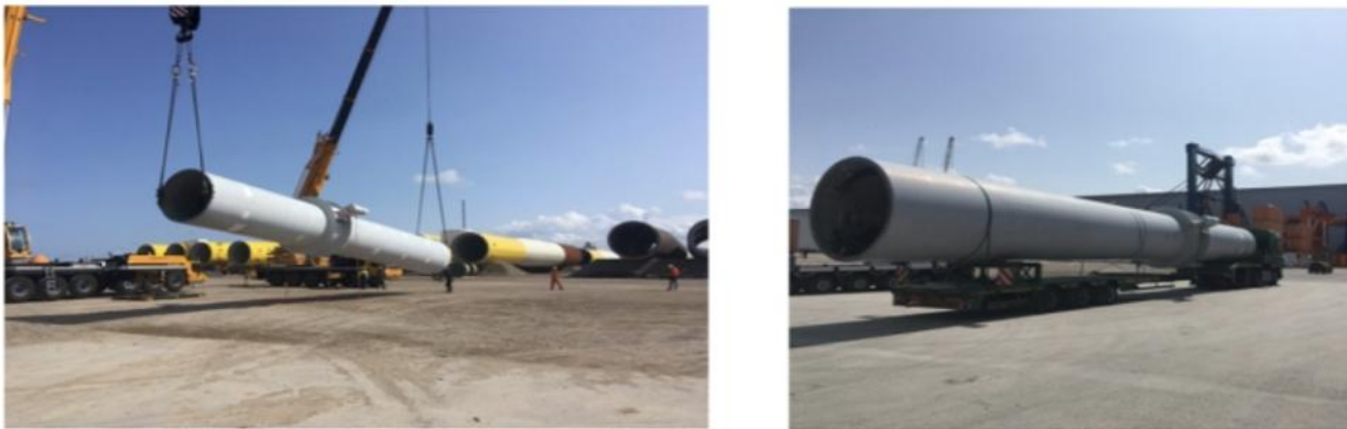
Figure 5: Installation of Upper Tower (DotPower, 2025)
