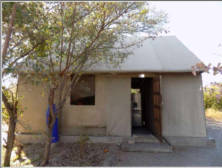
Figure 2: An example of the existing tented accommodation,
