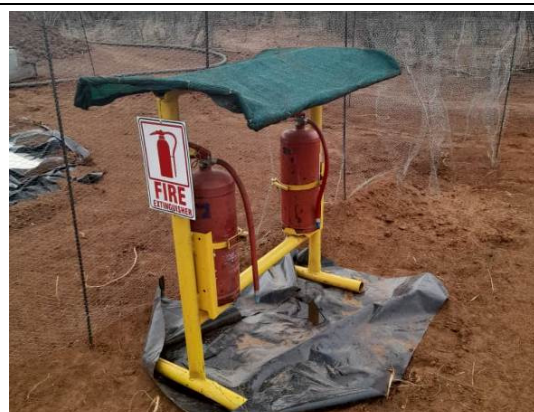
Photo 4-10 Firefighting equipment at drill site
