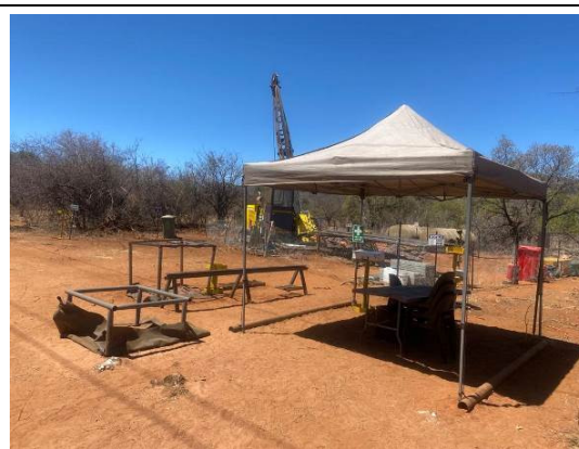
Photo 4-8 Core drilling site
