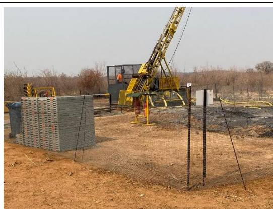
Photo 4-7 Core drilling site
