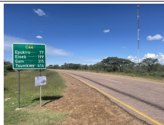
Photo 7-16 C44 trunk road (T14012)
