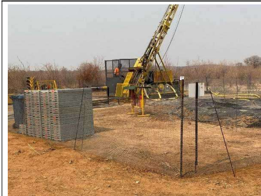
Photo 4-7 Core drilling site
