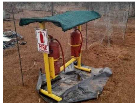
Photo 4-10 Firefighting equipment at drill site
