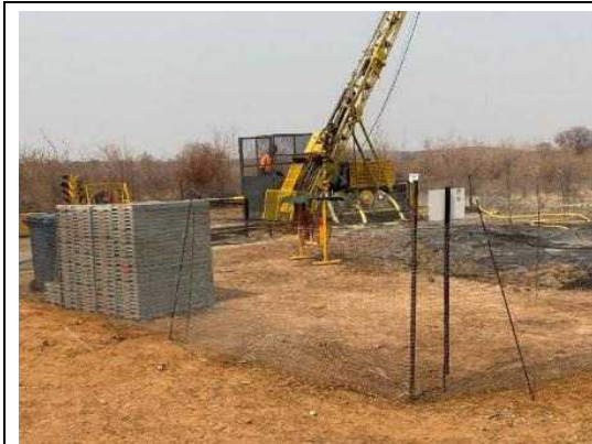
Photo 4-7 Core drilling site
